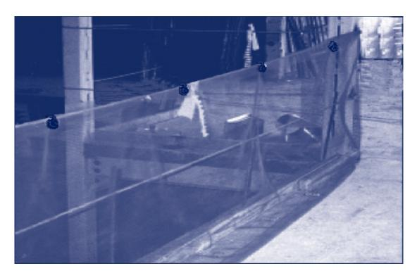
**GENERAL DESCRIPTION:** The system consists of 100 ft. long panels of bright safety orange, polyethylene mesh netting. "Easy Clips" and tie-down plates are also furnished in sufficient quantity for a complete installation. The system is available in heights of 48 inches and 66 inches from the floor. The 48 inch and 66 inch Vertical Debris Containment System is covered by U.S. Patent Numbers 4,815,562, 4,875,549, and 5,197,239. Other patents pending.
