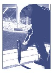
**WARNING:** The nail must penetrate fully so that the head is flush with the tie-down plate and the barrier is securely fastened to the floor.
